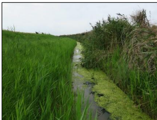
Photograph 6: Representative image showing the northern boundary ditch at the northern edge of the site.
