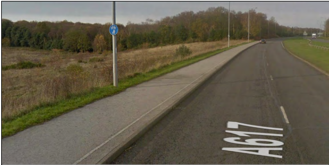
Figure 6: Footway on A617 Rainworth Bypass
